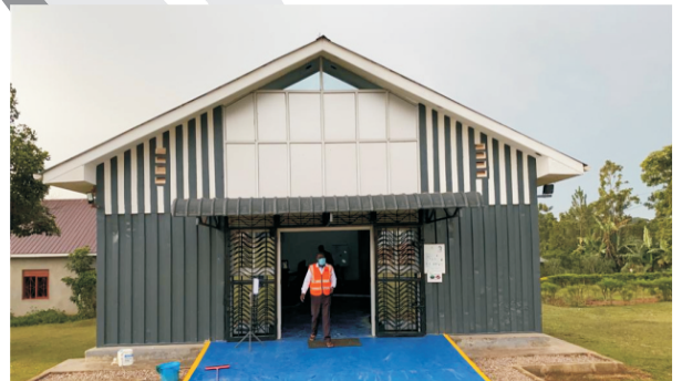
G-Tech Limited Offices
